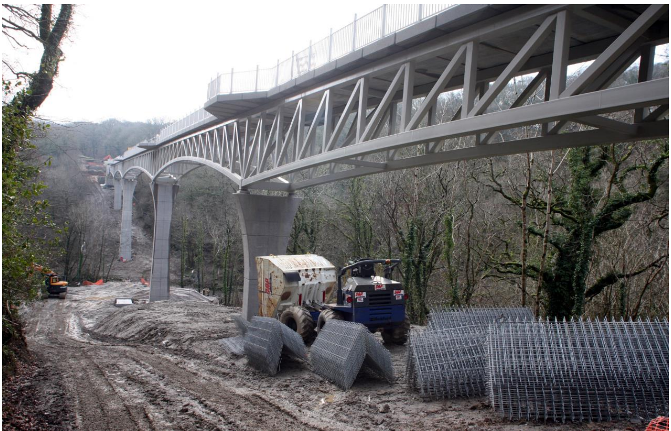
Gem Bridge (near Tavistock) Pedestrian / Cycleway 2013
